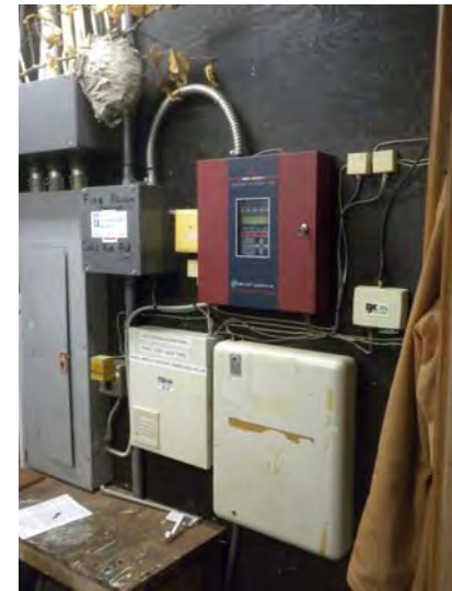
The central fire alarm control panel
