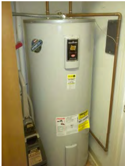
View of the electric domestic hot water tank serving the community building
