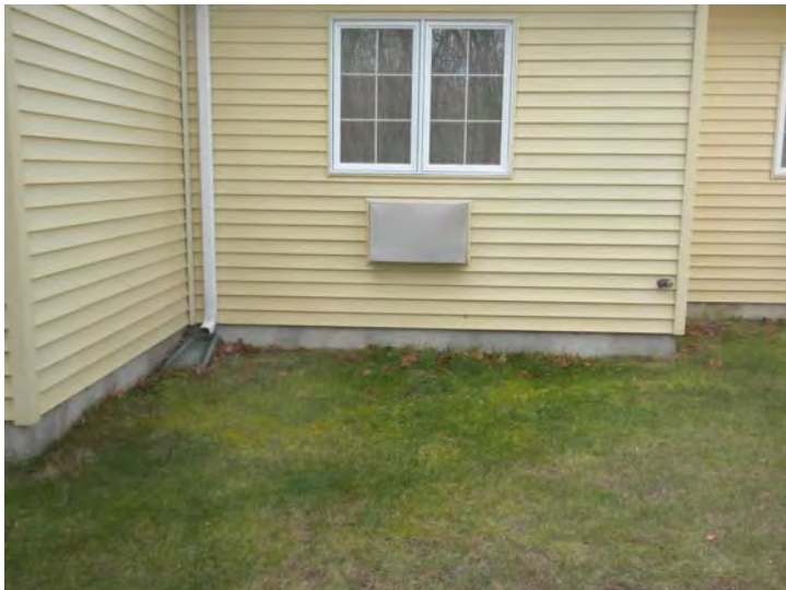
Air conditioning sleeves have exterior covers
