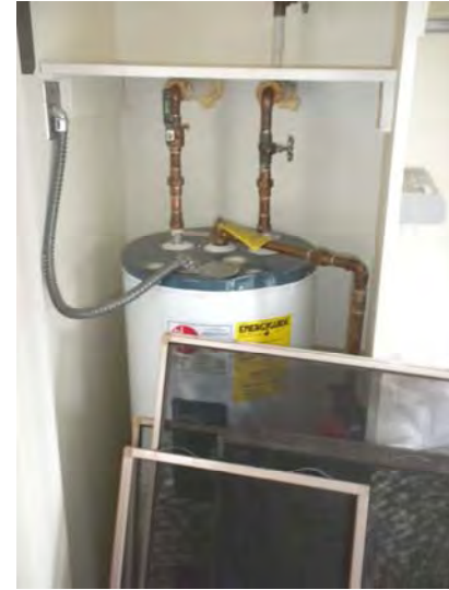
30-gallon electric domestic hot water tank
